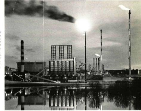
The tar sands processing plant at Fort McMurray in northeastern Alberta began operations in the fall of 1967, producing 45,000 bbl. of oil, 300 tons of elemental sulphur and 2,800 tons of coke daily from 110,000 tons of sand. Locked in the Athabasca tar sands is an estimated 600,000,000,000 bbl. of oil, an amount representing more than the combined reserves of all the oil fields in the world.
